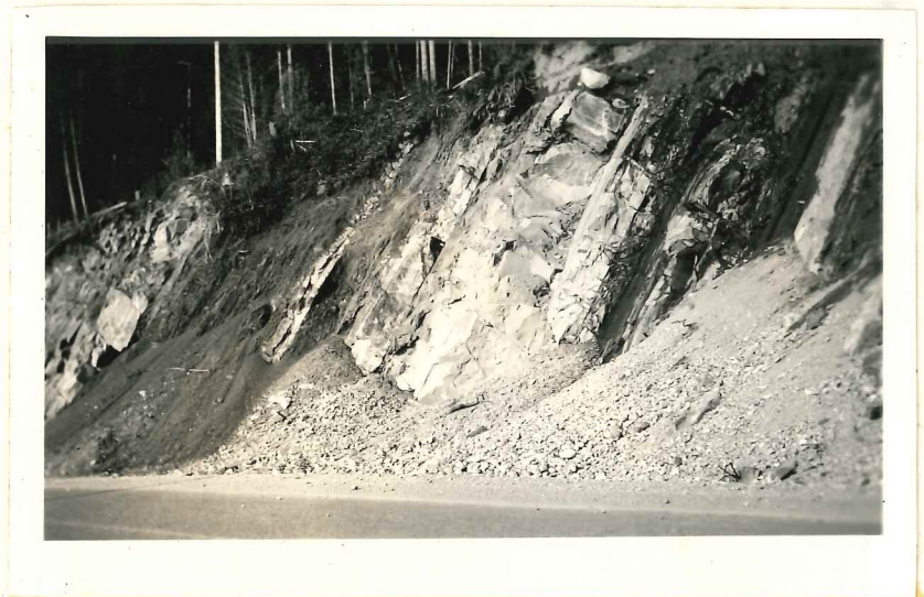
Fig. 2--Oligocene sandy shales and massive feldspathic sandstones outcropping on the Olympic Highway south of Lilliwaup.
