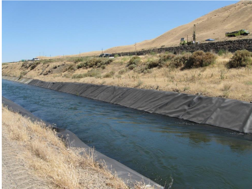
Figure 2: The KID Canal north of I-82 and the buttress. Cars on I-82 can be seen in the upper left of the photo. The shear-key buttress can be seen in the upper right with the WSDOT drilling crew during August 2013.
