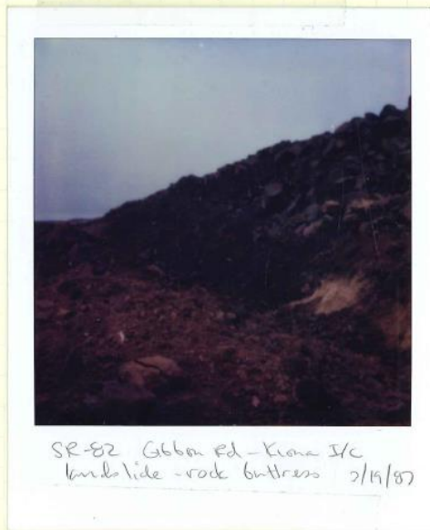
Figure 12: The second page of the March 20, 1987 Jenkins and Lowell memo showing annotated Polaroid photos of the shear-key buttress as it was being constructed. They argue that the buttress was not constructed to the specifications laid out by Todd Harrison. Specifically, in the photos they show that the buttress key is constructed above the planned grade. The buttress was not seated in the cut (ditch) at the bottom of the photos. Image courtesy of WSDOT via the Washington State Archives.
