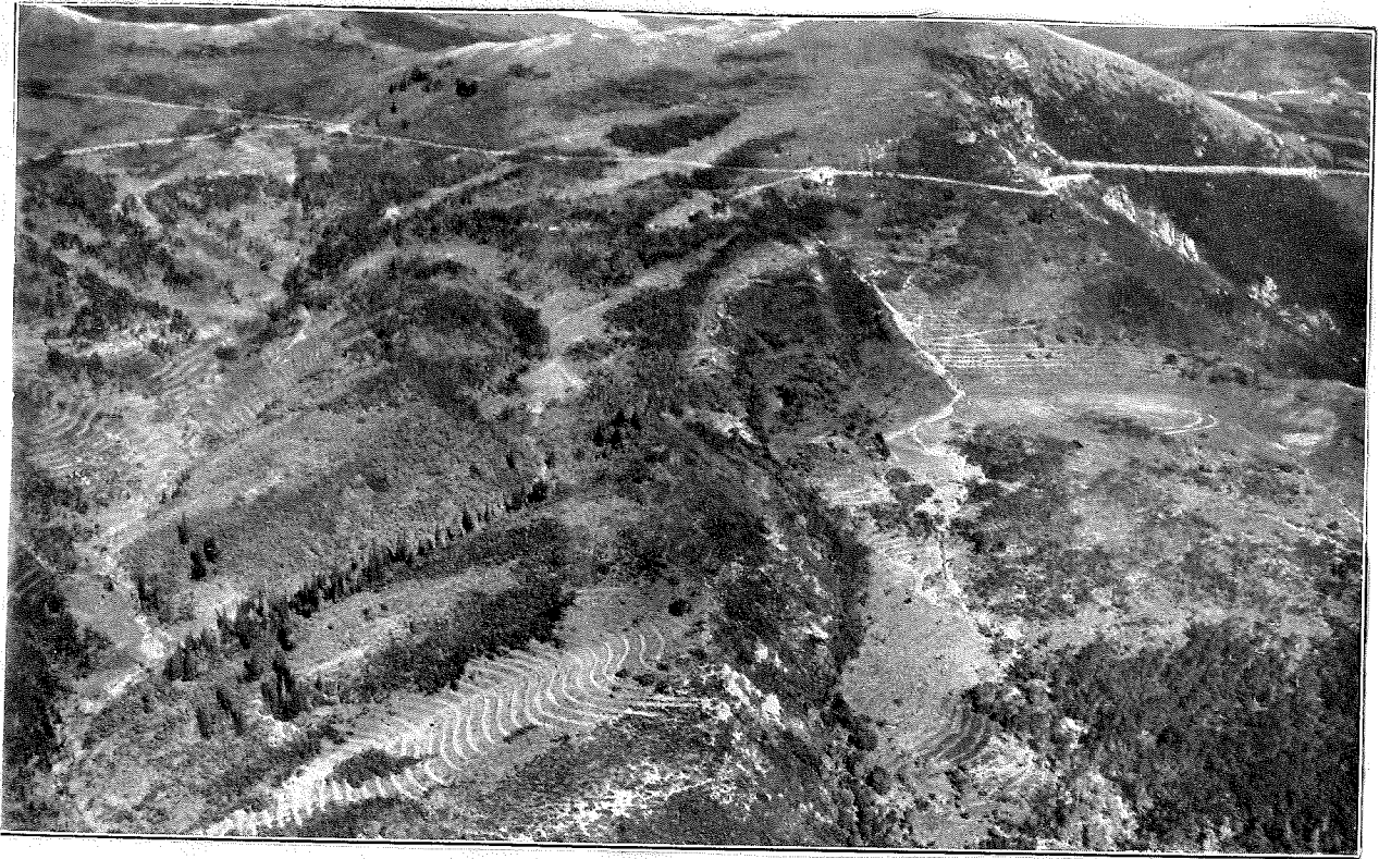
Plate # 5 Aerial View Of Contour-trenches
