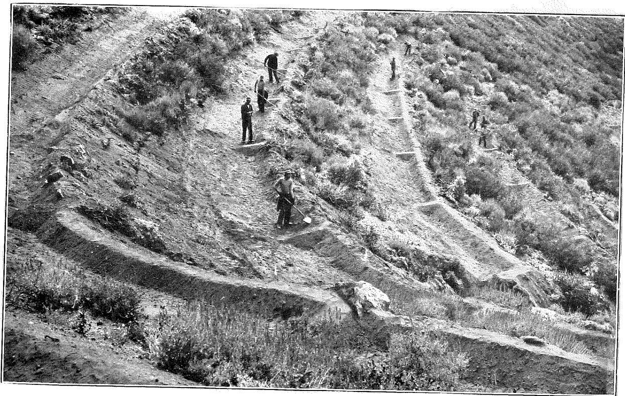
Plate # 6 Workers Finishing Contour-trenches
