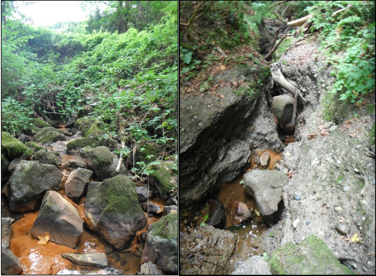
Figure 18. Photo of the upstream drain (left) and the slot-canyon.
