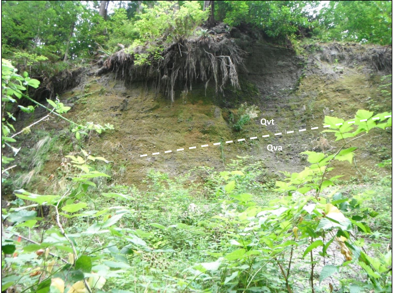
Figure 8. Landslide scarp and exposure of Qvt over Qva. The contact was interpreted where bedding associated with Qva was no longer observed.
