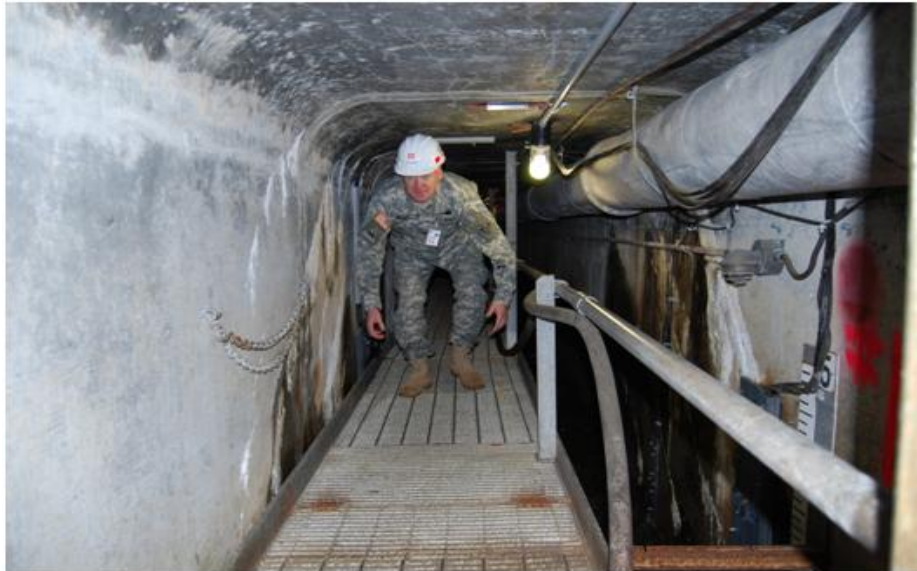
Figure 1-1: Relief Tunnel at Chief Joseph Dam.
